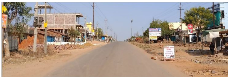
View of Kolar-Bhopal Road in the study area
