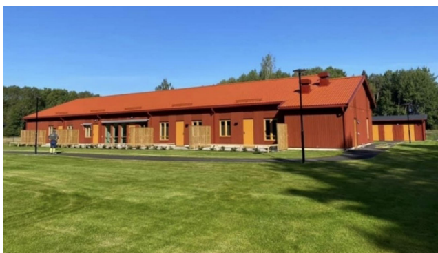
Figure 1 Overview picture of reference building
